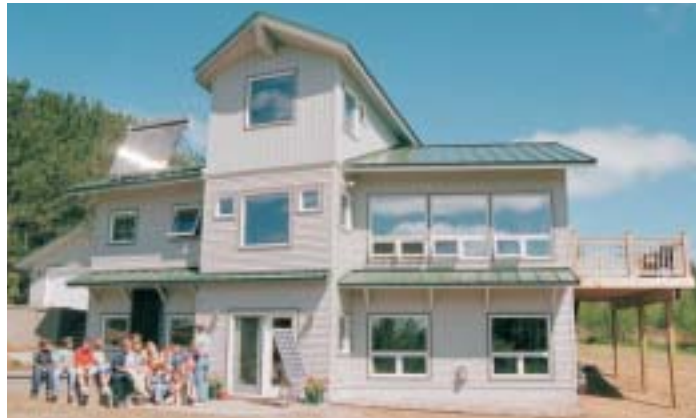
Thousands of people, many of them school children, have toured Minnesota Power's Millennium Star home, a super-energy-efficient house constructed in Duluth, Minnesota.
